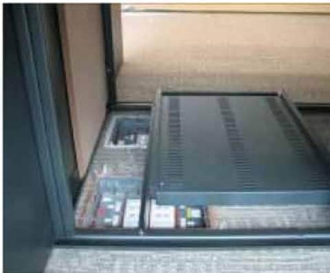
Floor box installation
